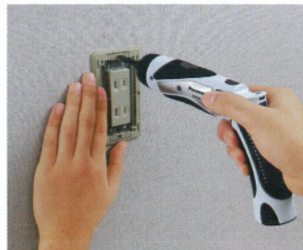
Installation of AC outlet
